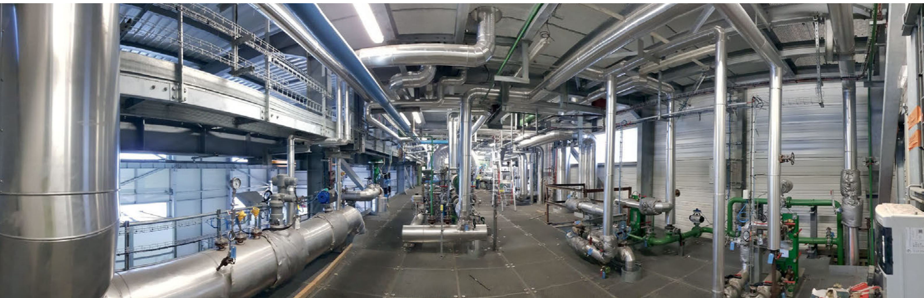
Tanks and exchangers
