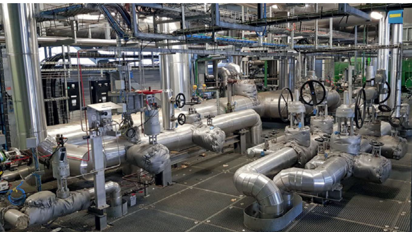
Cooling High and Low Pressure
