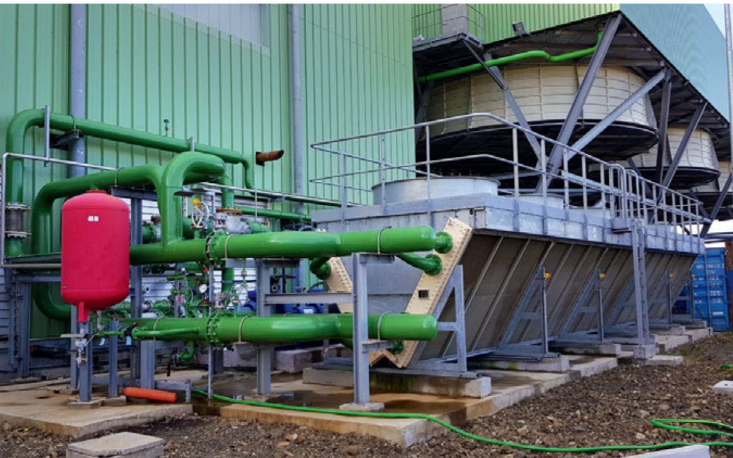
Cooling for Alternator
