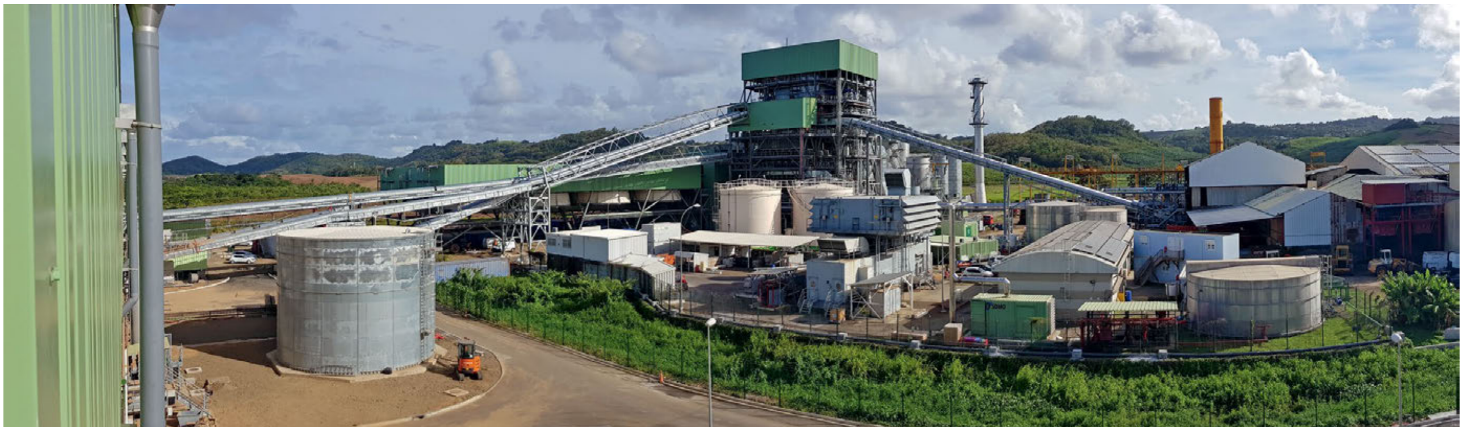
General view of Power Plant and Sugar Plant on April 6, 2018
