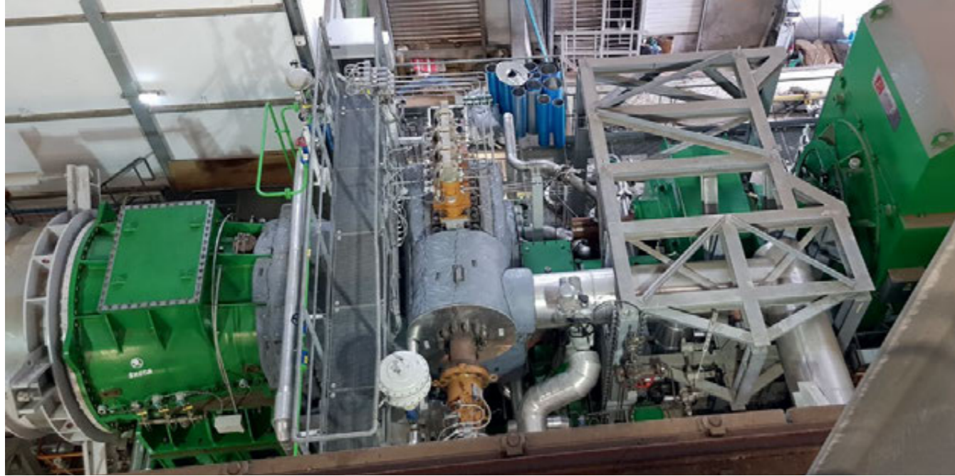
Turbine and Connection of High Pressure Steam Piping line
