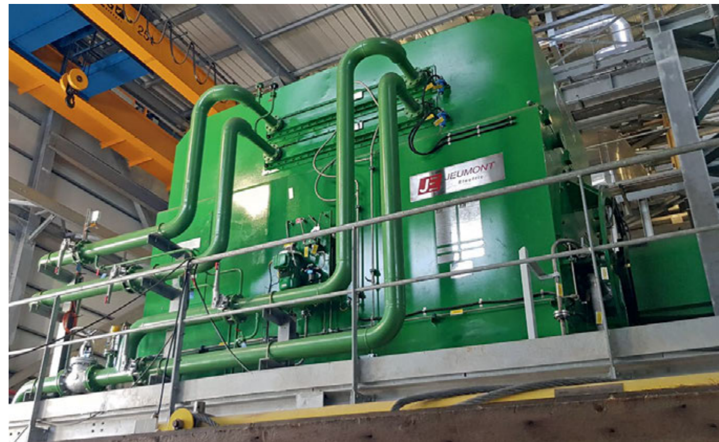
Cooling for Alternator
