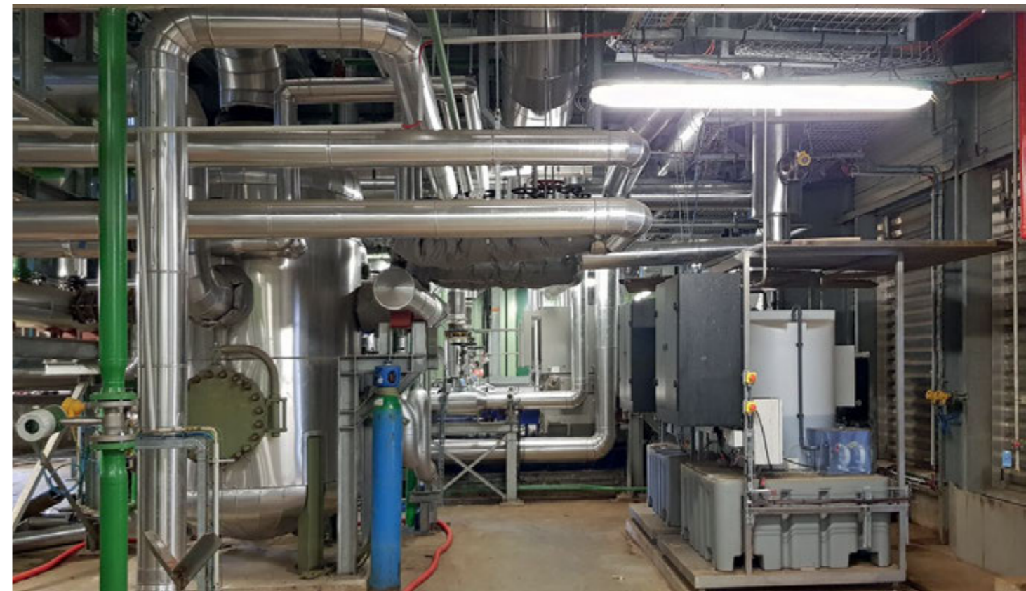
Chemical tanks on skids
