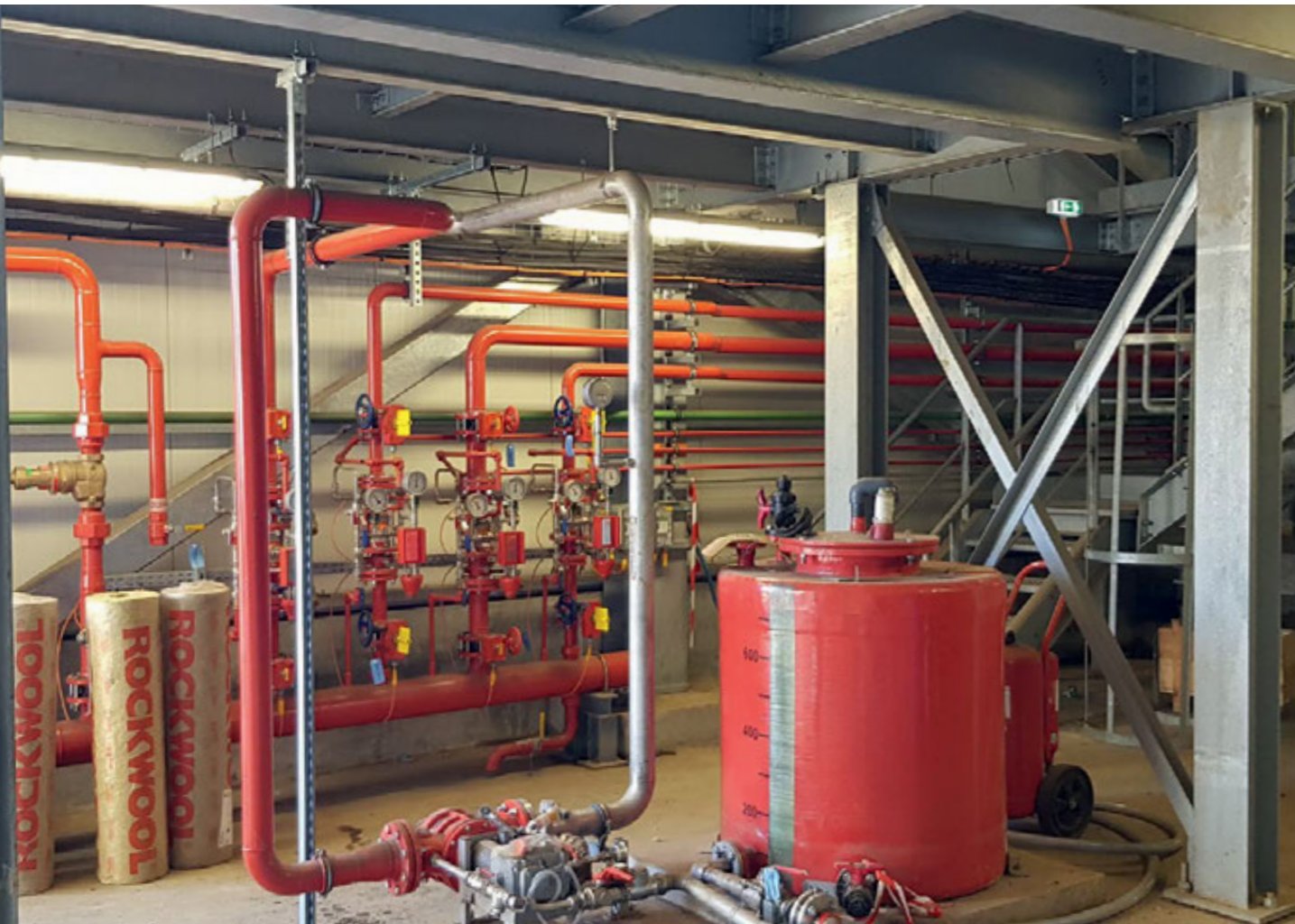
Fire networks and pipes for Engine's Room
