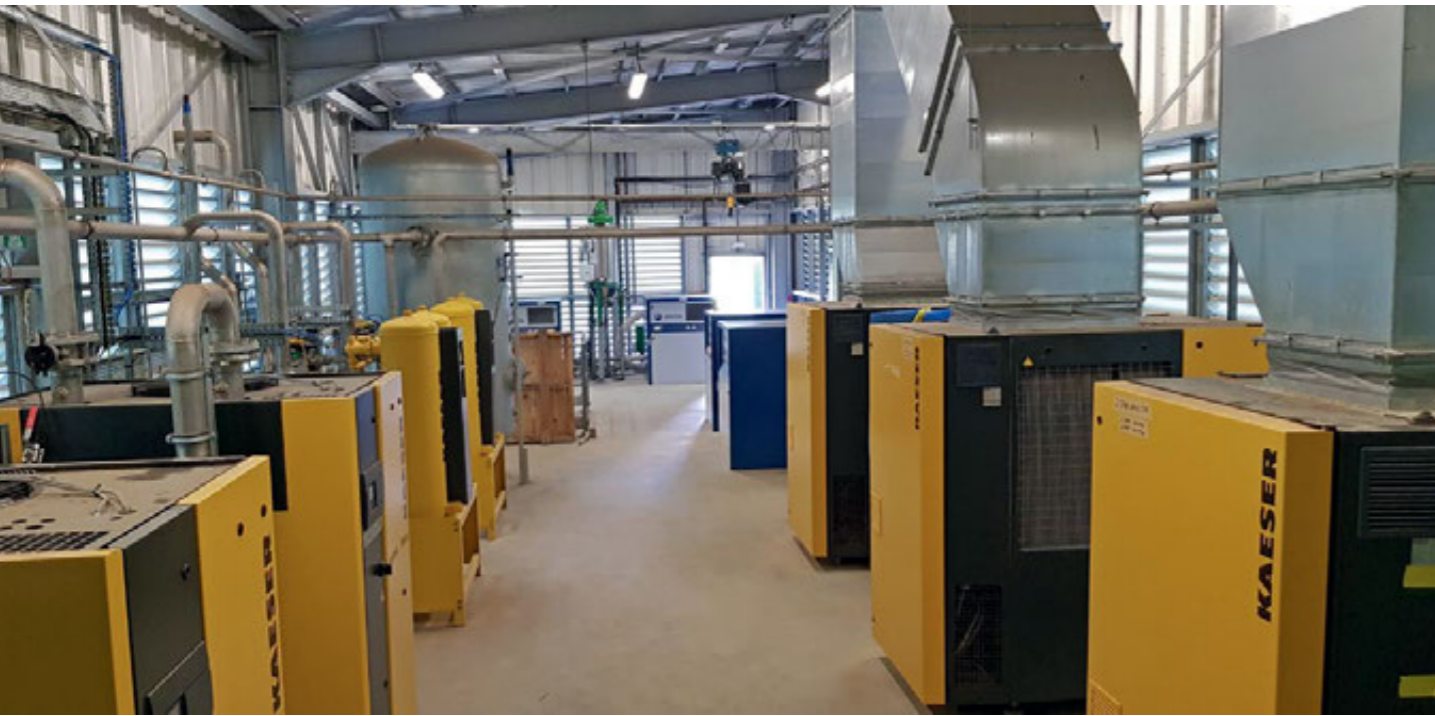
Pipes for fumes exhausting compressors
